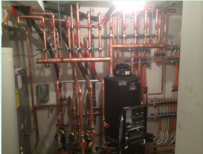
3 Ton geo with hybrid air source heat pump water heater
